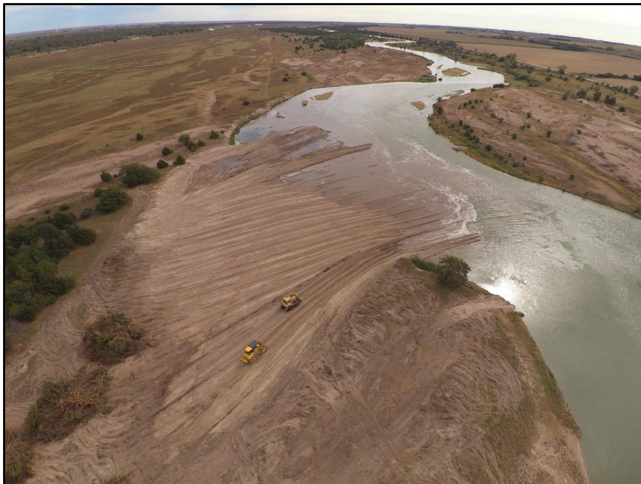
Figure 1.6 Construction of 2019 Sediment Augmentation Project (42,300 yd 3 ).
